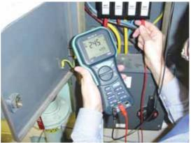
Checking the circuit continuity by multimeter
